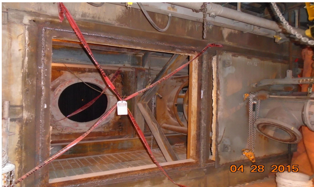
Boiler preparation to add new gas burners
