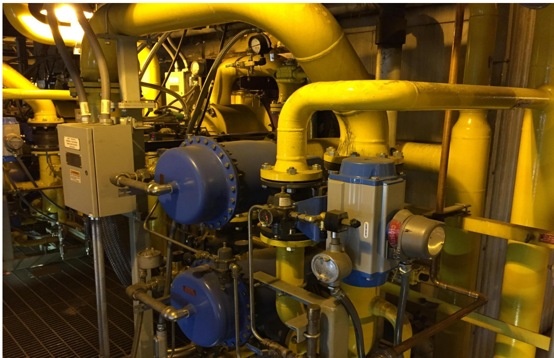
Installing new gas burners
