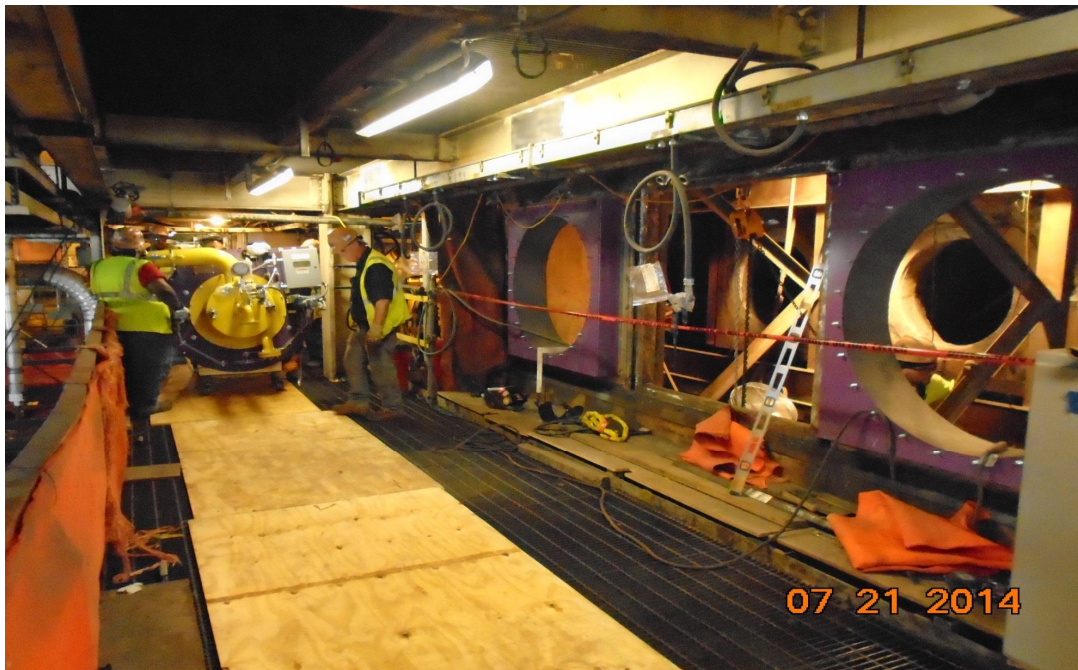
Installing new gas burners
