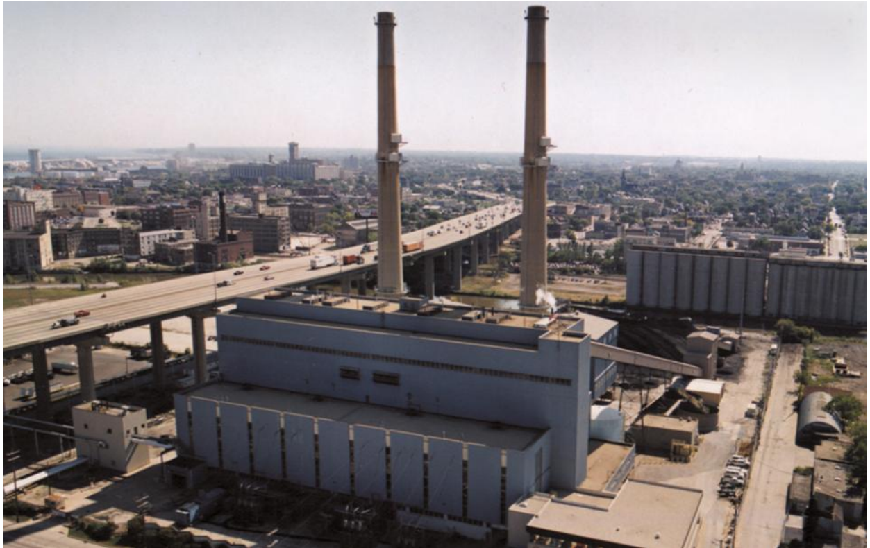
We Energies Valley Power Plant, Milwaukee, Wisconsin
